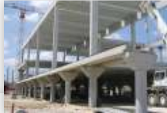
Precast Concrete Installation
